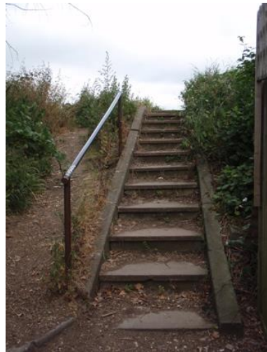
Steps at Common Rise entrance
